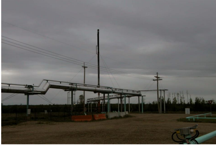
Figure 7: Flare piping between FKOD and Flare Stack
